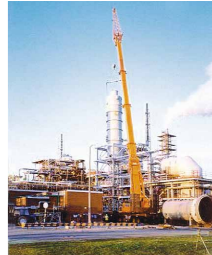
Assembly of a SO 2 -scrubber for 60,000 Nm 3 /h
