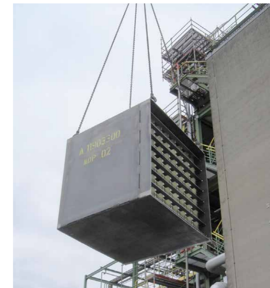
Assembly of a catalytic converter equipped with catalytic ceramic honeycombs
